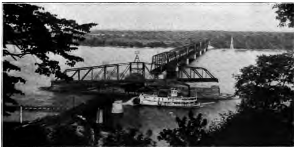
Photo by F. M. Fulls. DOUBLE TRACK RAILWAY BRIDGE OF THE C. B. & Q. R. R., OVER THE MISSISSIPPI AT BURLINGTON, IA., SHOWING THE DRAW OPEN AND STEAMBOAT PASSING THROUGH. The flood plain on the Illinois side is seven or eight miles wide.
